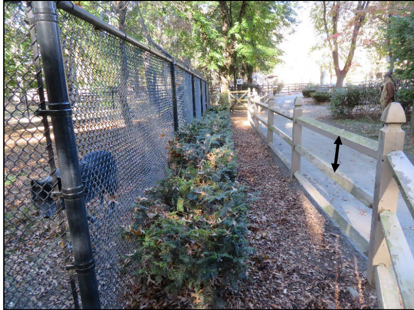
Figure 5: Public barrier at a grey wolf exhibit scoring 2 out 3. Gaps (arrow) between rails of this post and rail fence could allow an unattended child easy access to the primary enclosure.
