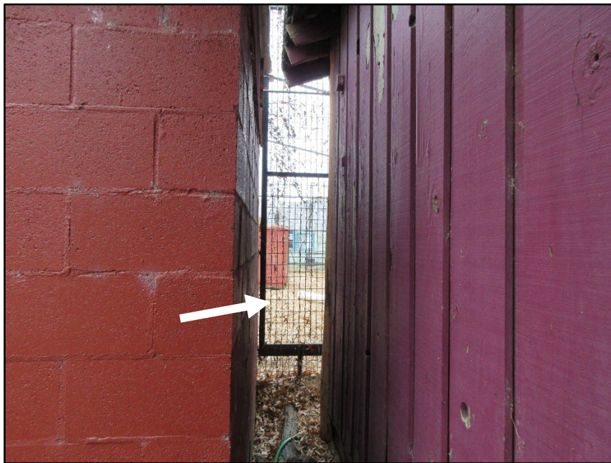
Figure 3: Lion exhibit with an unprotected gap between the lion house and a reptile house allowing direct access to the primary enclosure. Arrow indicates the wall of the primary enclosure.
