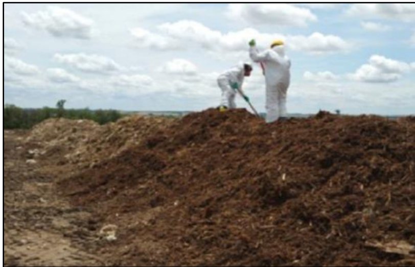
Figure 13. Capping the Windrow
