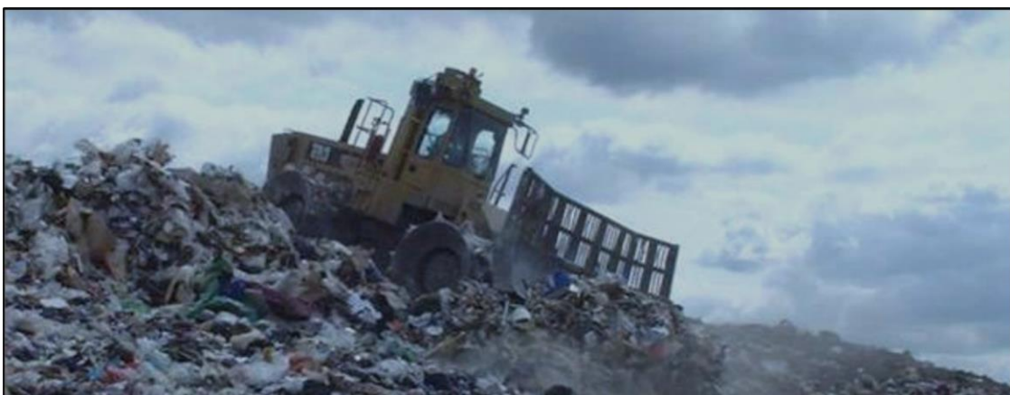
Figure 4. Compacting Deposited Waste
