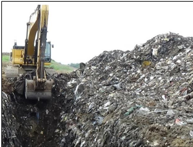
Figure 12. Excavating the Trench
