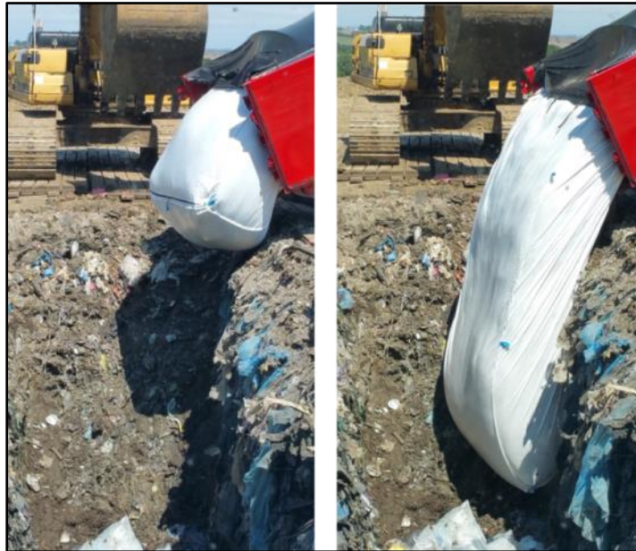
Figure 13. Liner Sliding Into the Trench
