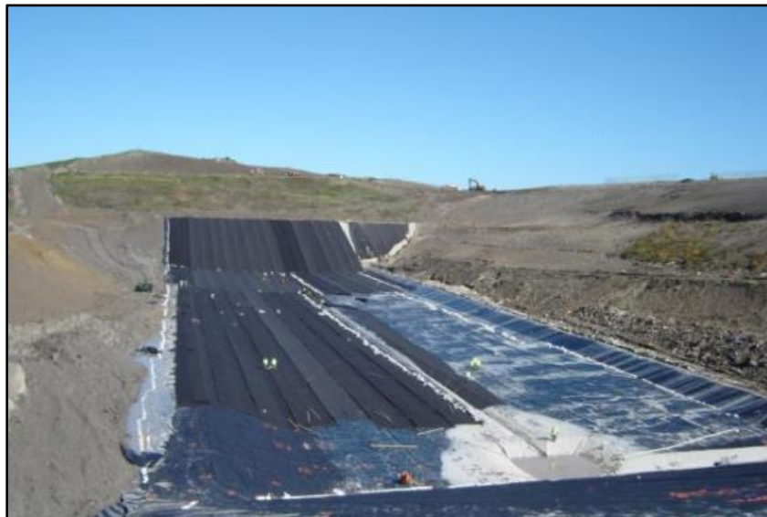
Figure 5. Prepared Landfill Site
