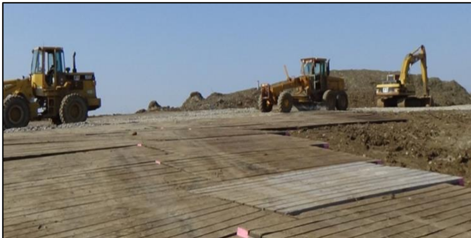
Figure 11. Prepping the Landfill Roads
